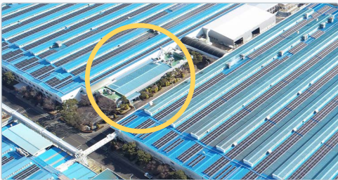
Solar Power Installation at Jigok Plant 2
